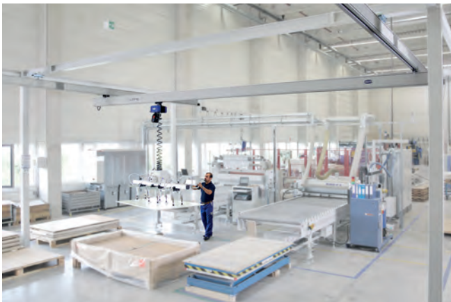
Aluminum single bridge crane system with conductor line and vacuum lifting device VacuMaster Comfort destacking wall panels
